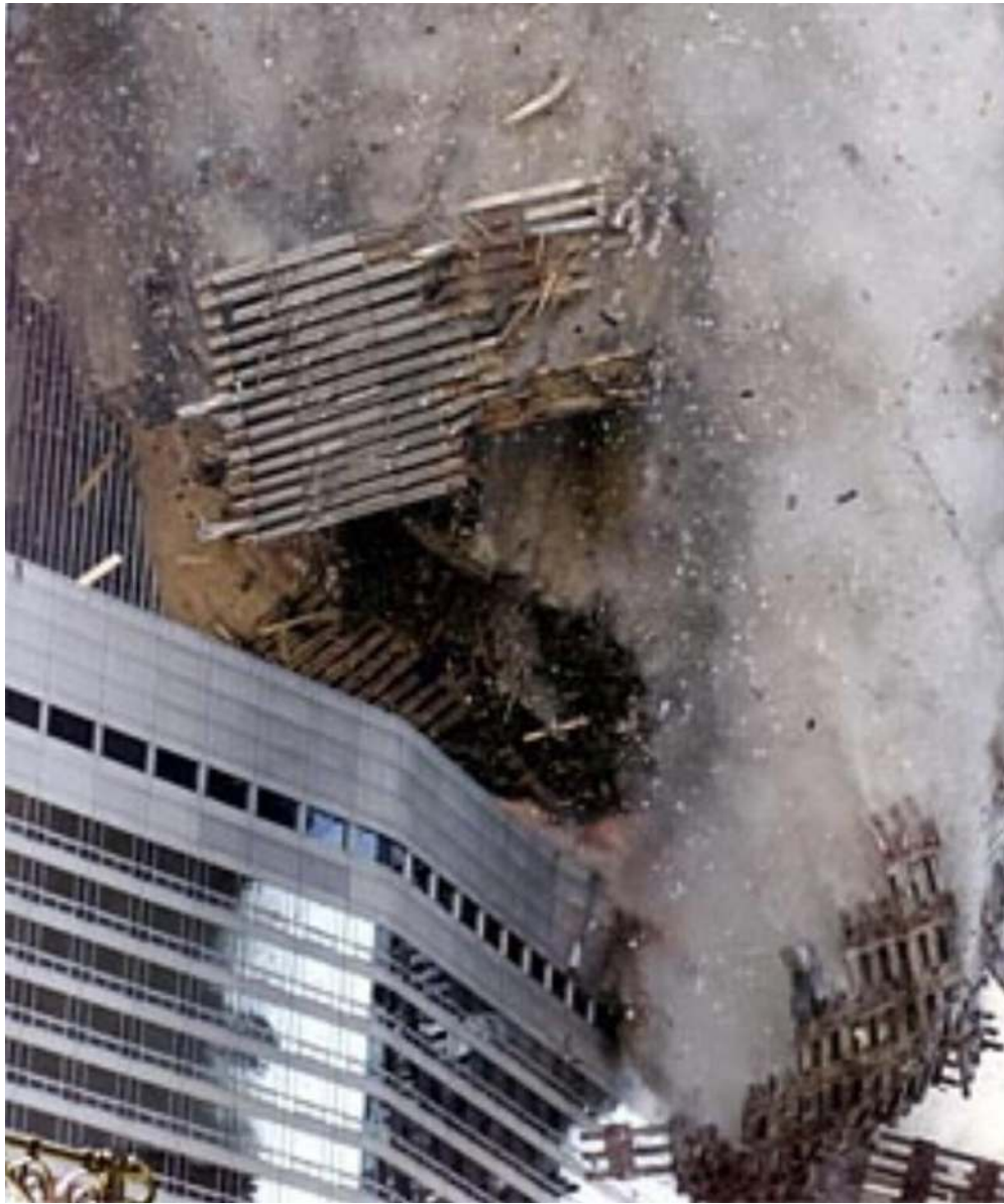
The towers collapsing
