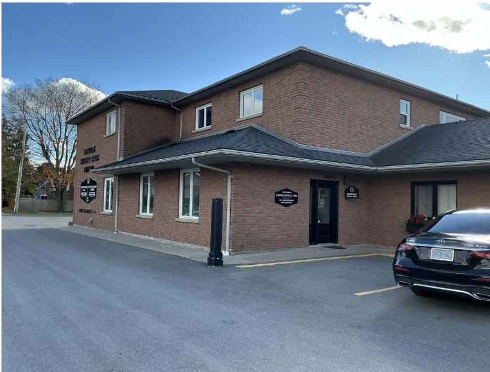
The Elmvale office on Stone Street fifty years later and with a second floor
